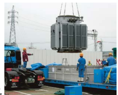
Transporting PCB containing devices
